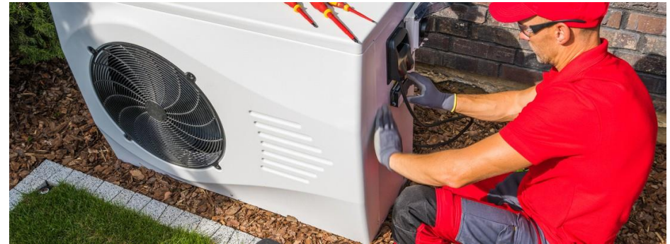
Pictured: A contractor installing a heat pump in a garden.
