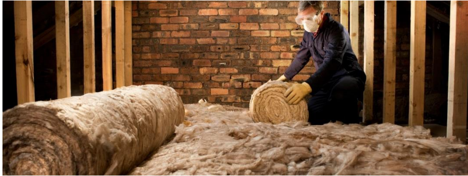
Pictured: A contractor installing loft insulation.
